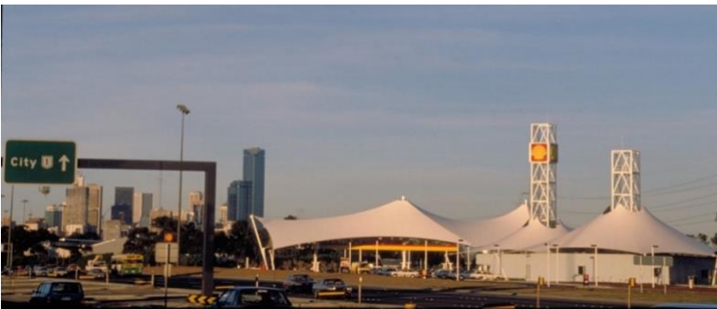
Figure 55. The completed structures at the southern site, looking east (Source: Spacotech collection).
