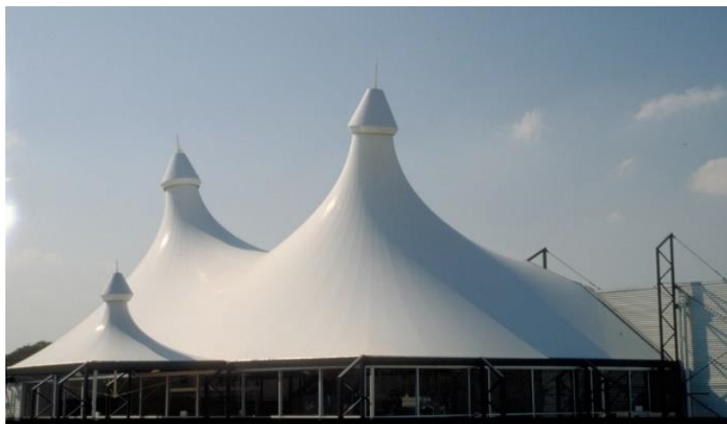
Figure 27. The Keysborough Golf Club driving range roof (Source: Spacetech collection).
