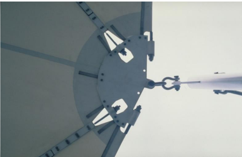
Figure 59. Detail of the completed structures (Source: Spacetech collection).
