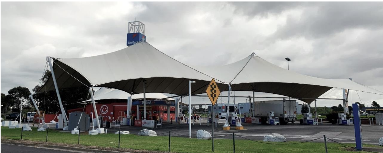
South service station site, 2 West Gate Freeway, Port Melbourne (GJM Heritage, August 2021).
