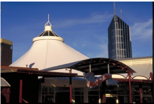
Figure 68. Roof over the food court, Queen Victoria Market (demolished 2022) (Source: Peter Kneen collection).
