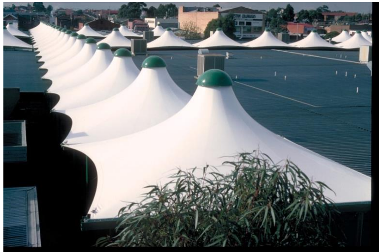
Figure 26. Top view of the Preston Market redevelopment membrane structures (Source: Spacotech collection).
