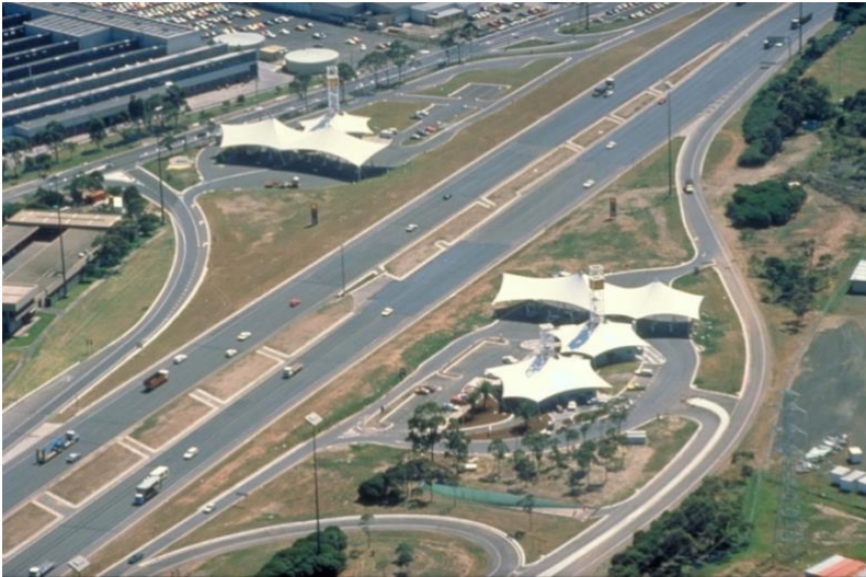
Figure 53. Aerial view of the completed sites (Source: Spacotech collection).
