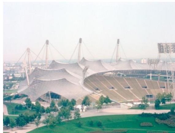
Figure 5. Munich Olympic Stadium cable net structures by Frei Otto (Source: Peter Kneen collection).
