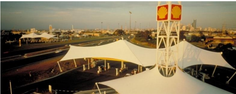
Figure 54. The completed structures (Source: Spacotech collection).
