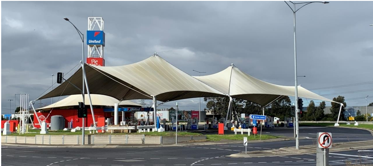
North service station site, 1 West Gate Freeway, Port Melbourne (GJM Heritage, August 2021).
