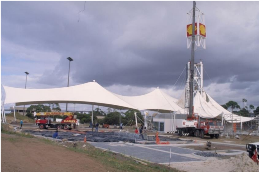
Figure 49. Crane in the course of erecting the structures (Source: Spacetech collection).
