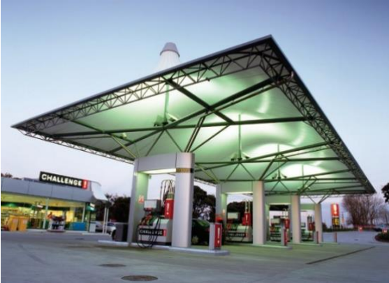
Figure 43. A Challenge service station canopy, c1999 (Source: Structurflex, 'Challenge Gas Service Station').
