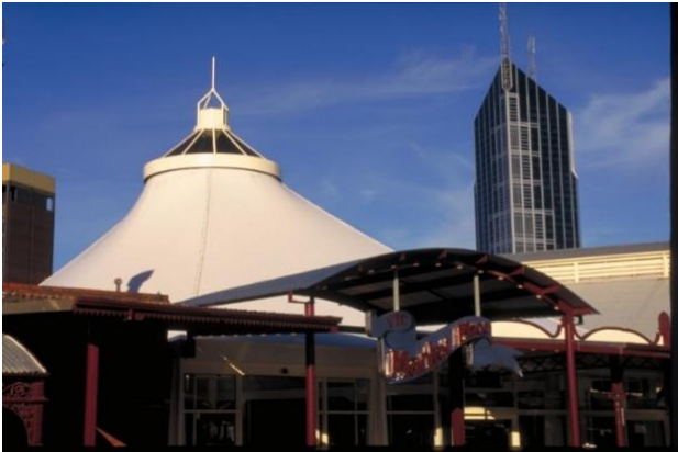
Figure 30. Roof over the foodcourt, Queen Victoria Market (demolished early 2022) (Source: Peter Kneen collection).
