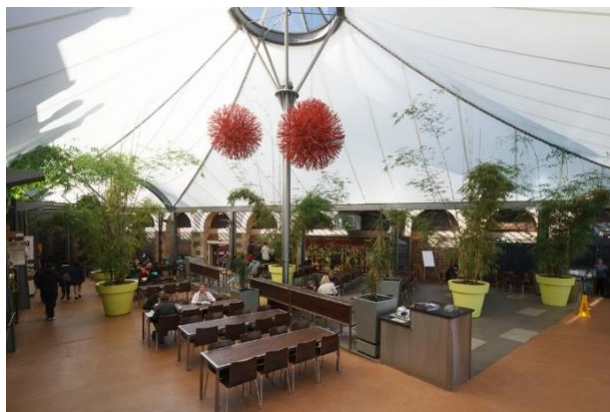
Figure 31. Interior of the Queen Vic Market foodcourt roof (demolished early 2022) (Source: ACLA Consultants).
