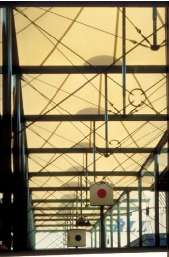
Figure 25. Structures to the arcades, Preston Market redevelopment (Source: Spacetech collection).
