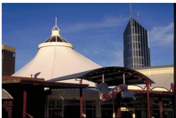
Figure 68. Roof over the food court, Queen Victoria Market (demolished 2022) (Source: Peter Kneen collection).
