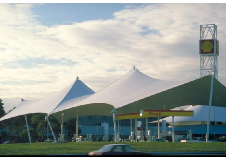
Figure 56. The completed structures (Source: Spacotech collection).
