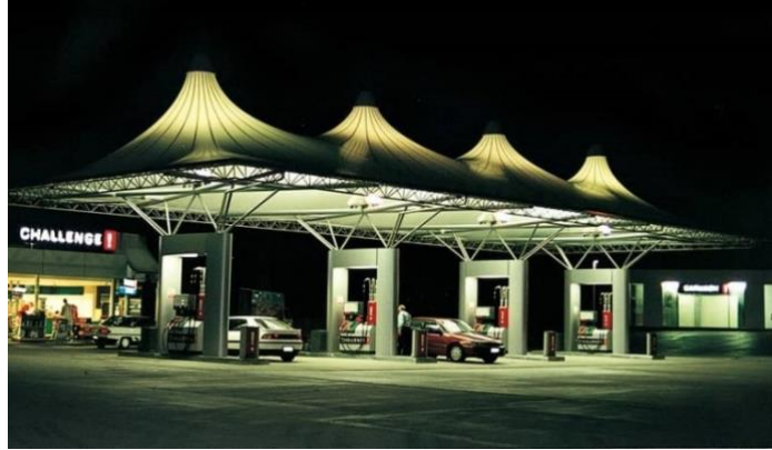
Figure 44. A Challenge service station canopy, c1999 (Source: Shelter-Rite Architectural fabrics).
