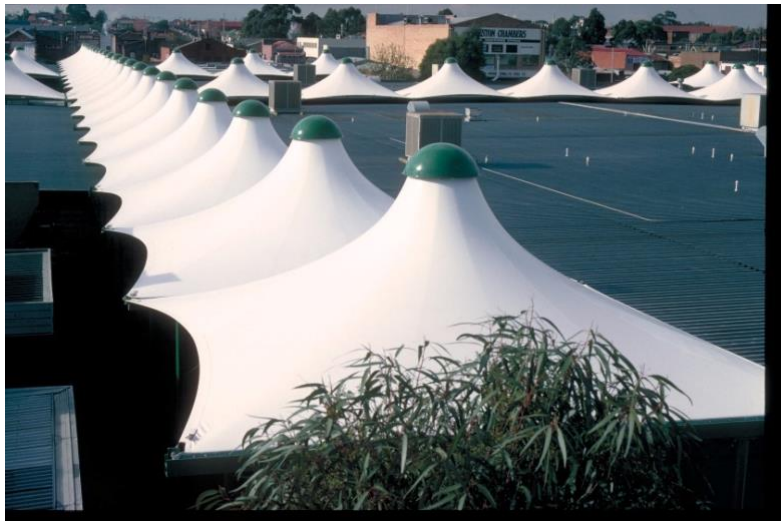
Figure 26. Top view of the Preston Market redevelopment membrane structures (Source: Spacetech collection).
