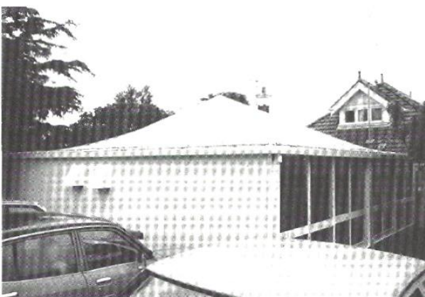
Figure 6. The 'Art House' roof structure at Ivanhoe Girls' Grammar, 1982 (Source: Picker & Sedlak 1982:31).
