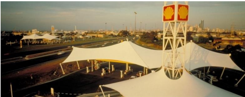
Figure 54. The completed structures (Source: Spacotech collection).
