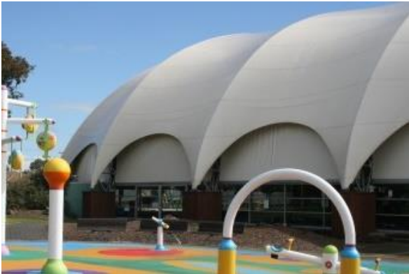
Figure 8. The Norlane Olympic Pool roof structure in 2015 (Source: Ausleisure).
