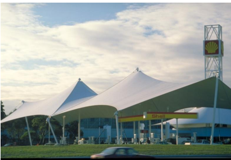
Figure 56. The completed structures (Source: Spacotech collection).
