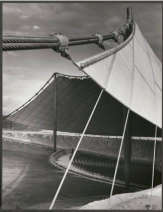
Figure 66. The Sidney Myer Music Bowl structure in 1959 (Source: Mark Strizic, via Docomomo Australia).
