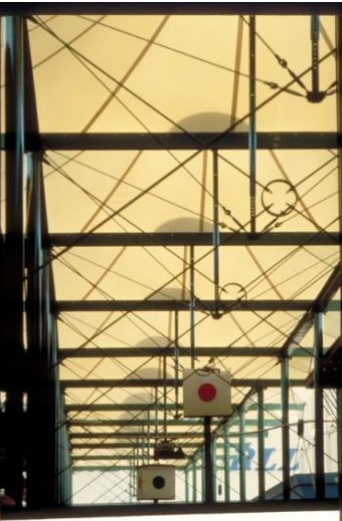
Figure 25. Structures to the arcades, Preston Market redevelopment (Source: Spacotech collection).
