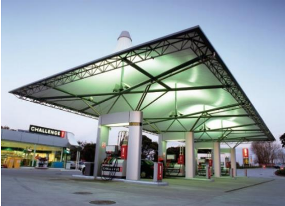
Figure 43. A Challenge service station canopy, c1999 (Source: Structurflex, 'Challenge Gas Service Station').
