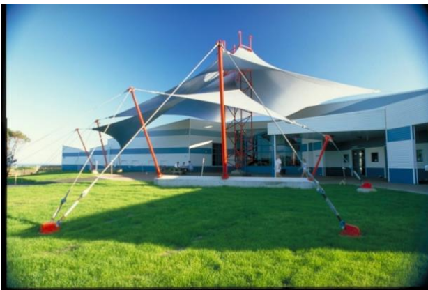
Figure 22. The entrance structure at the Penguin Parade visitor centre (Source: Spacetech Collection).
